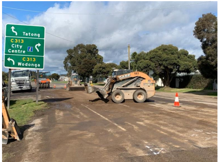
Figure 19: BRCC road construction projects
